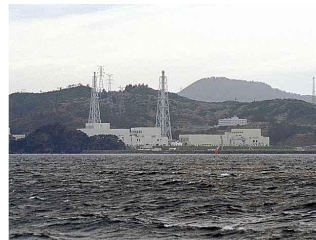
Onagawa nuclear power station
